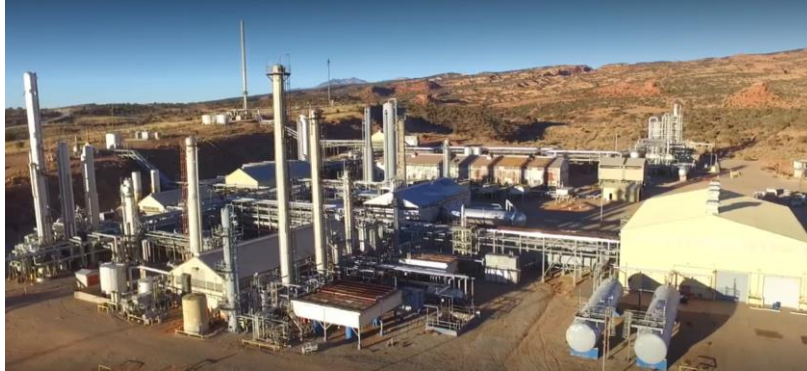
Paradox Resources Lisbon Valley Gas Processing Plant.
