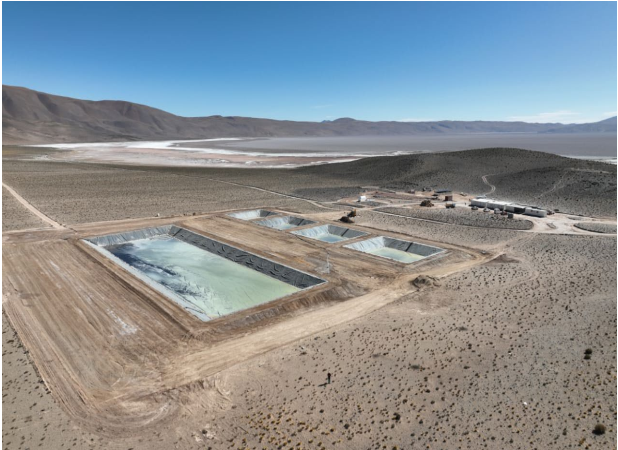
Figure 7: Aerial view of S1 pond filling with brine with camp and the Hombre Muerto salt flat in the background
