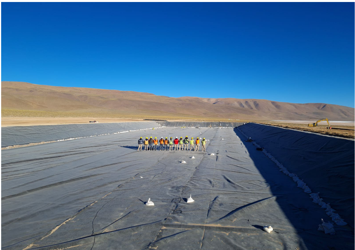
Figure 6: Evaporation Pond S1 Construction
