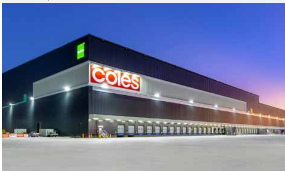
Redbank Motorway Estate, Brisbane, Australia
