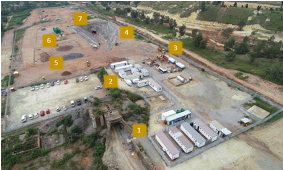
IMAGE 6: COMPLETED INFRASTRUCTURE AT QALA SHALLOWS
