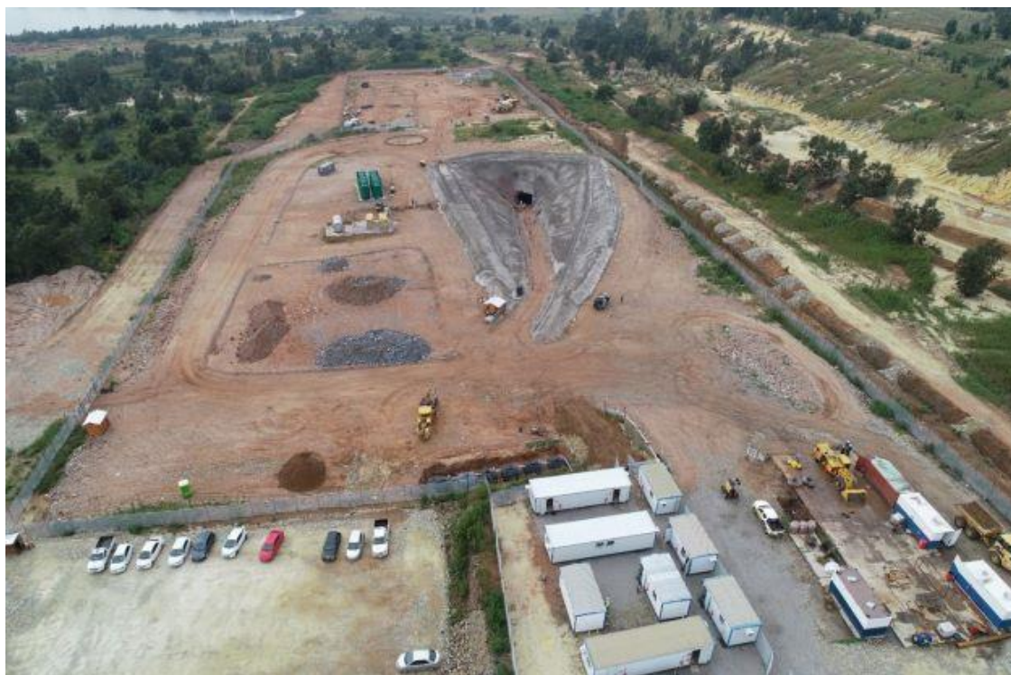
IMAGE 1: COMPLETED INFRASTRUCTURE AT QALA SHALLOWS
