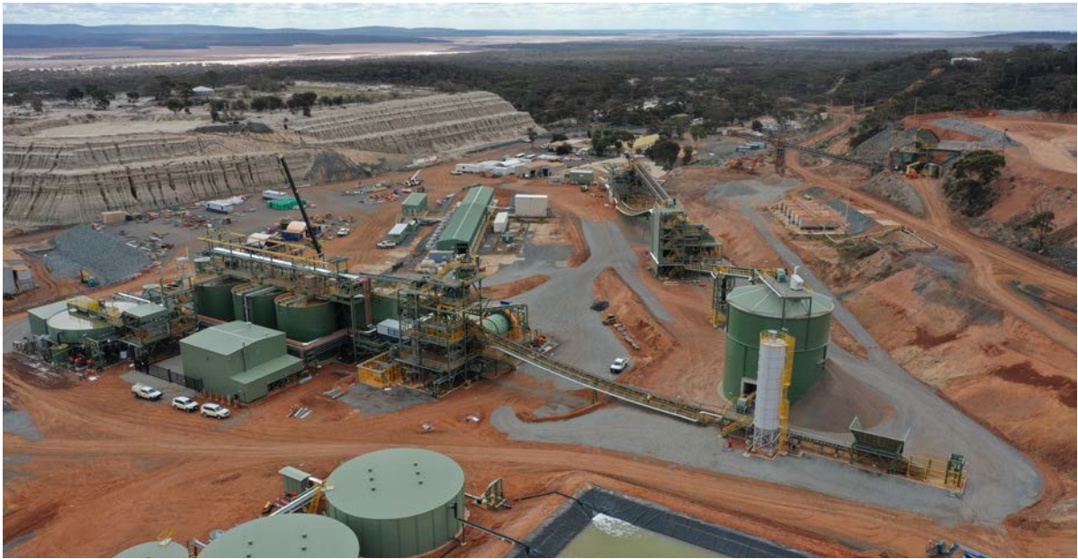
New processing plant undergoing commissioning in September 2022.
