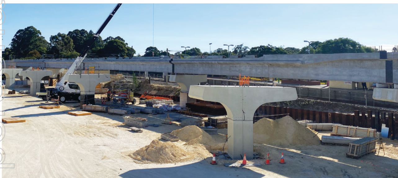
Columns, headstocks and beams installations at Evolve Bayswater Train Station
