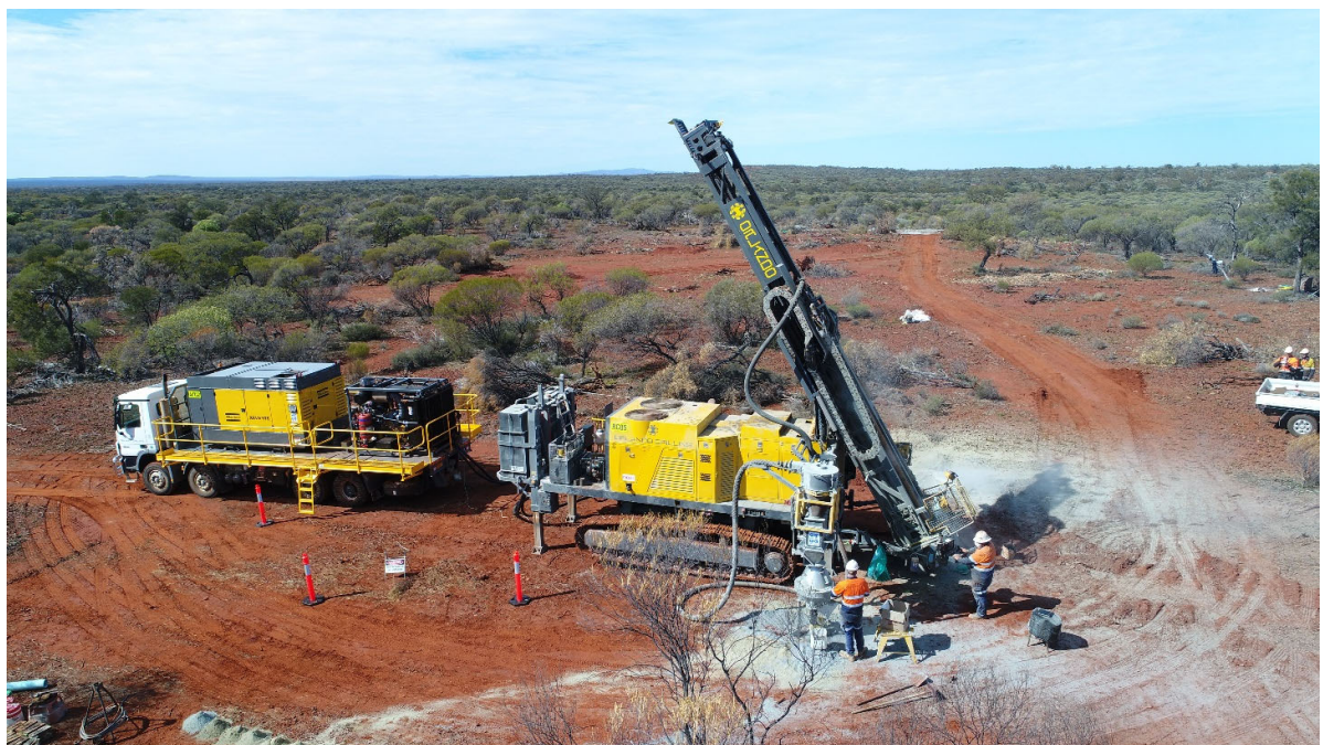
Picture 1: Orlando Drilling rig completed all drilling at Smokebush Gold Exploration Project.
