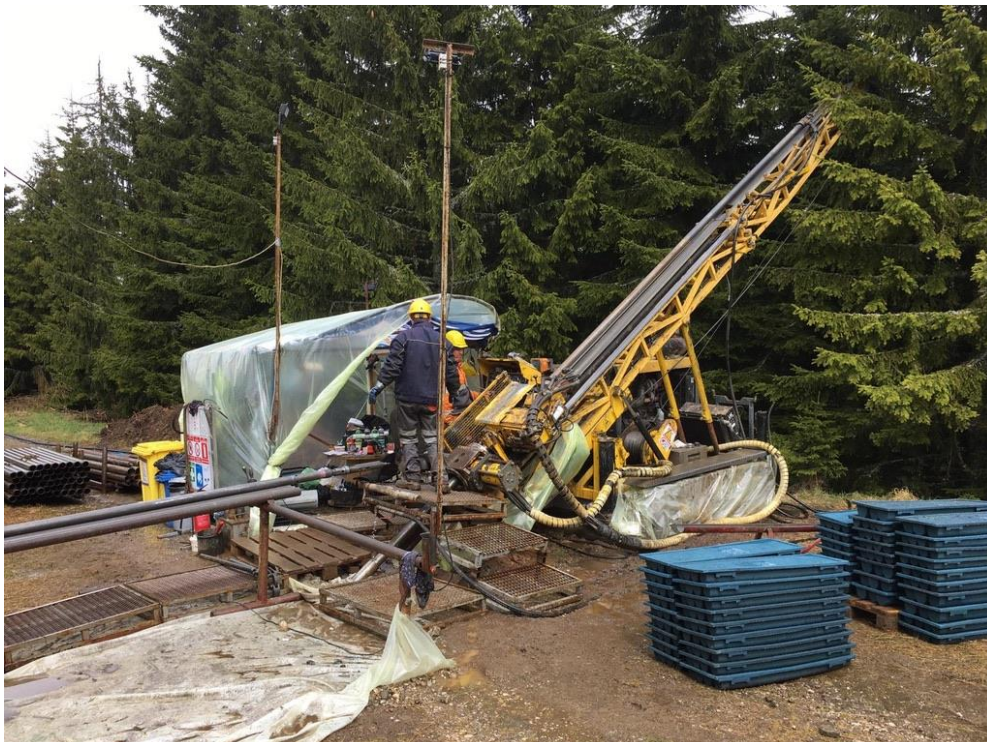
Figure 1 – Drill rig 1 in operation
