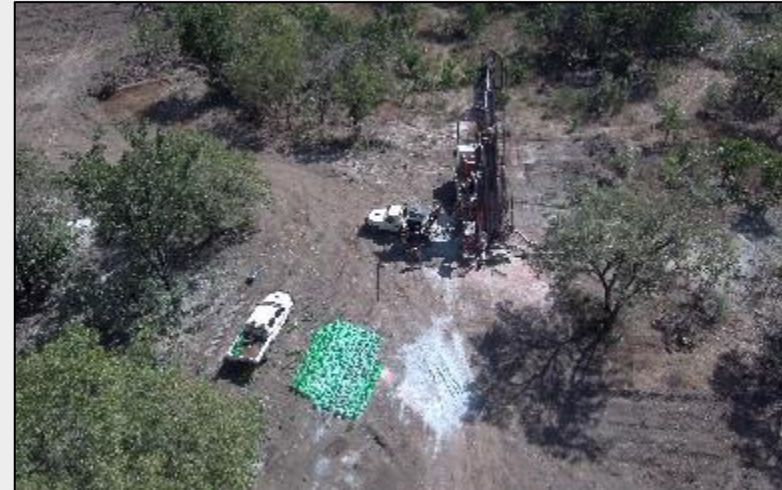
Aerial of drill rig
