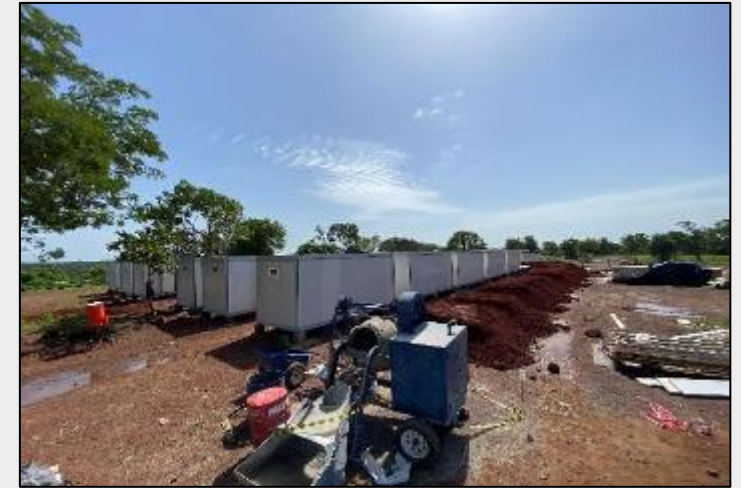
Construction of camp facilities
