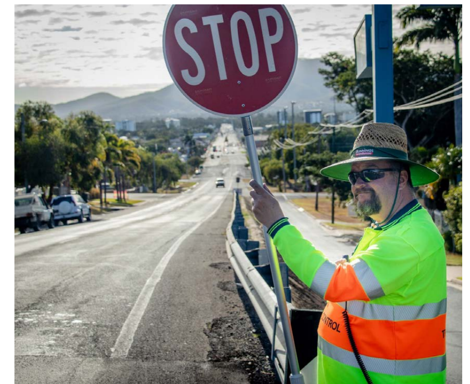
East Coast Traffic Control
