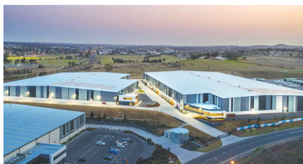
Ingleburn Logistics Park, NSW
