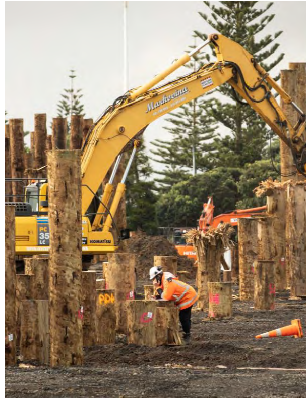
Foundation piles for the Transport Hub
