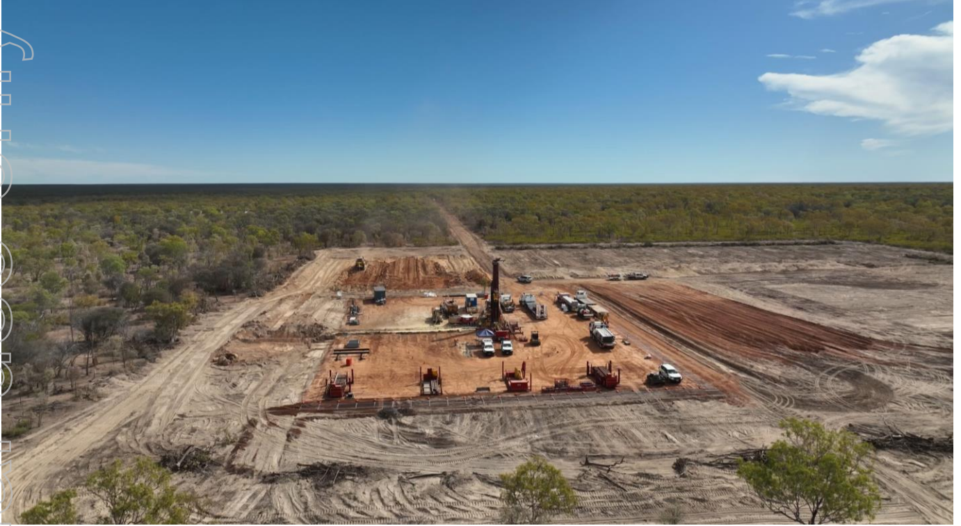
Figure 2: Pad construction and water bore activities within EP 136.
