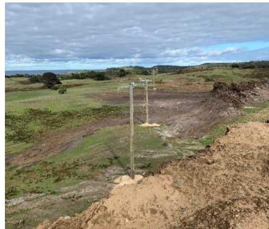
Figure 4 - Overhead Site Power Connection from King Island Grid
