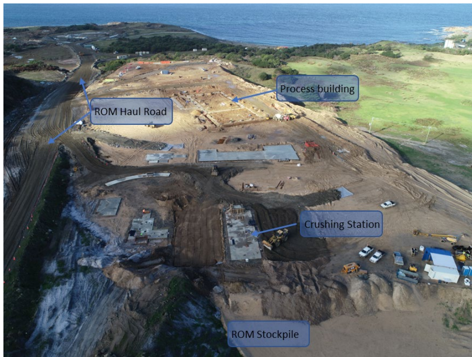
Figure 1 - Process Plant Construction Activities
