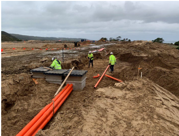
Figure 3 - Installation of Electrical Pits and Conduits for Process Plant
