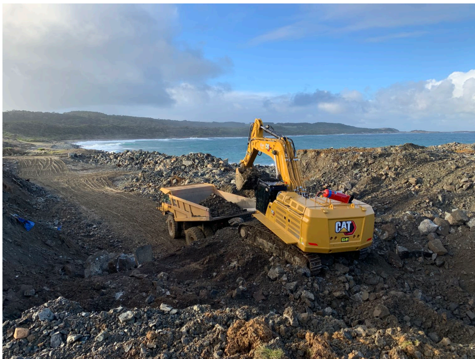
Figure 2 - Recovering Road Base Material at Dolphin Tungsten Mine
