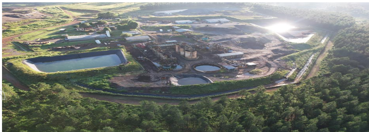
Figure 1 Panoramic view of TGME Processing Plant, Workshops and Tailings Dam
