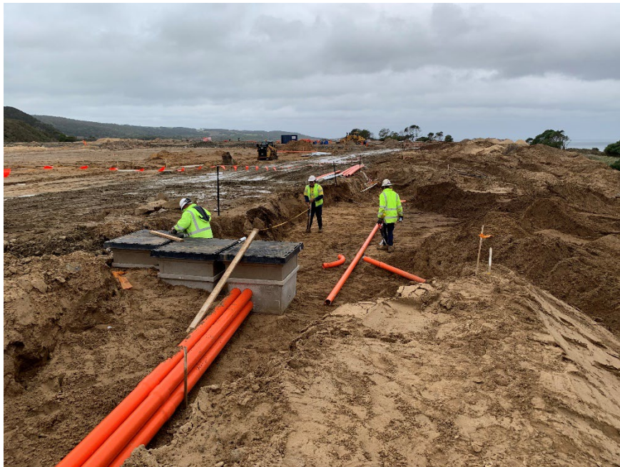
Figure 3 - Installation of Electrical Pits and Conduit
