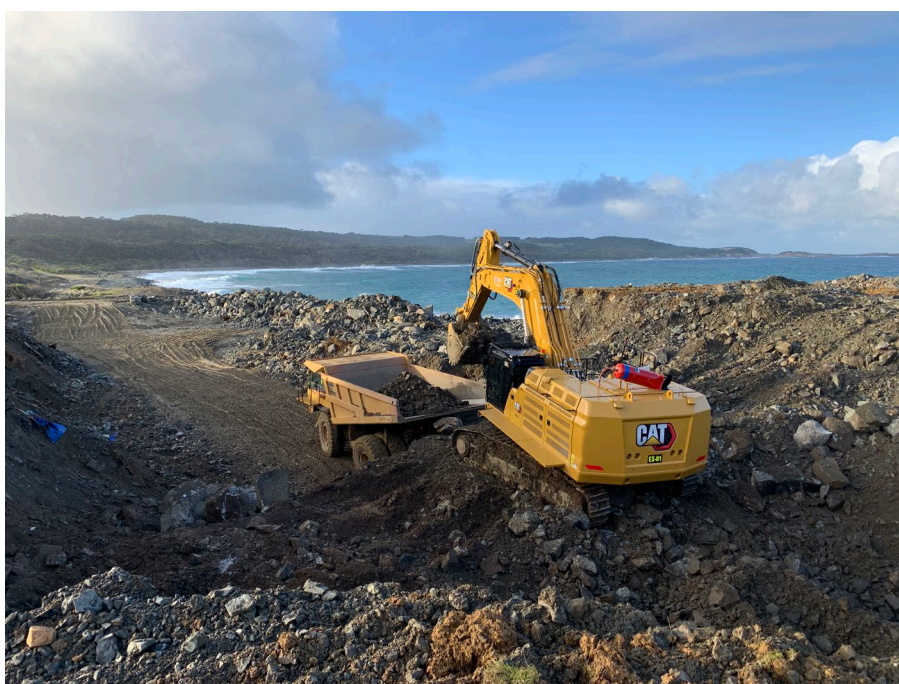
Figure 2 - Recovery of road base material for Internal Roads
