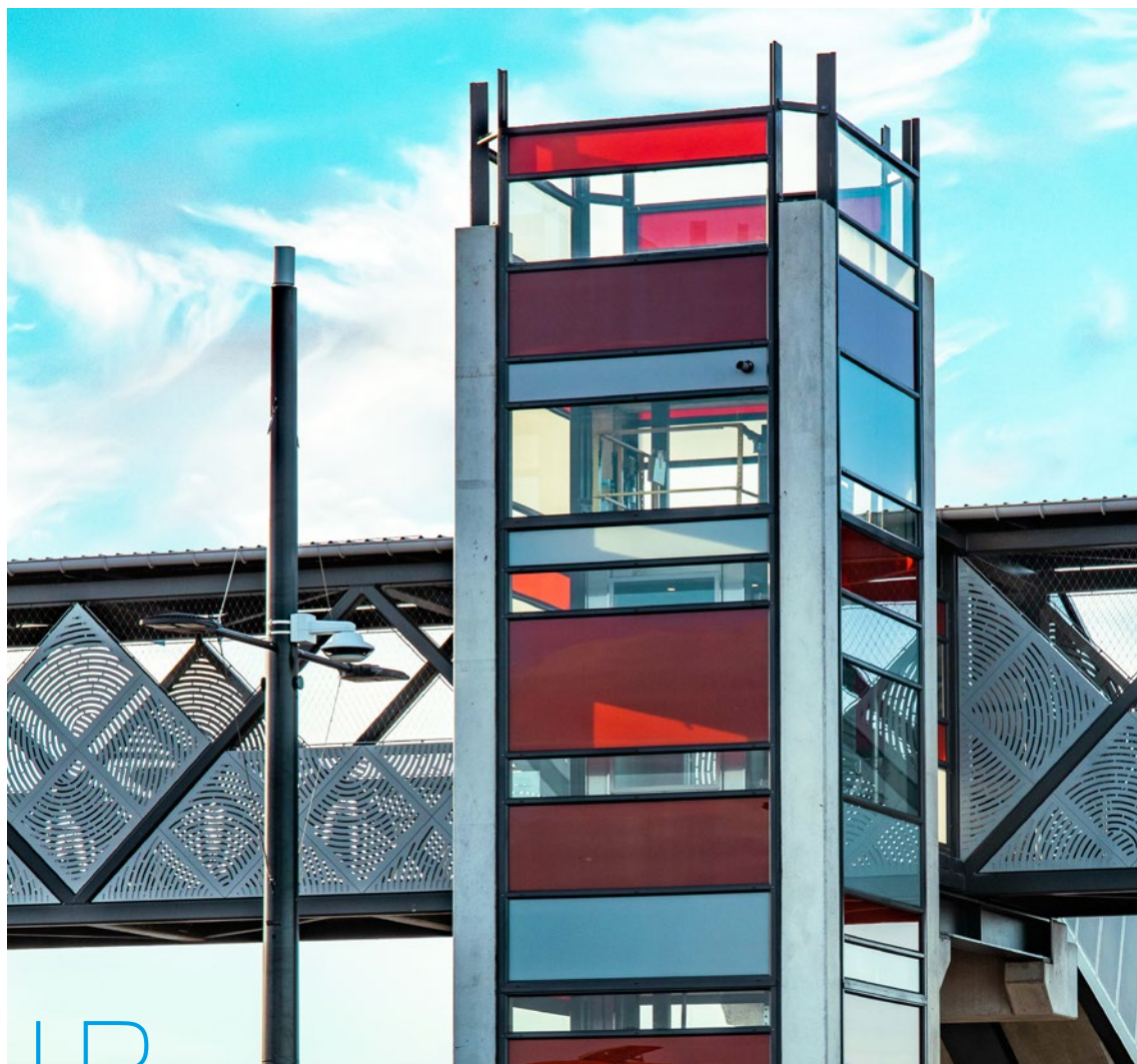
Transport Hub Lift Shaft, Laminated Toughened Safety Glass with RED Pet Film
