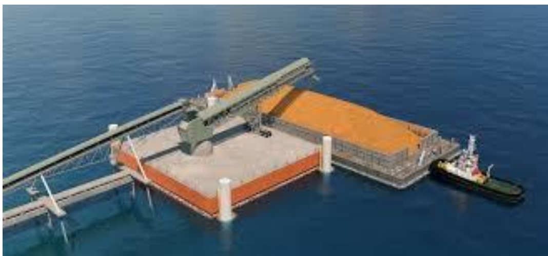
Figure 20: Typical radial telescopic barge loader
