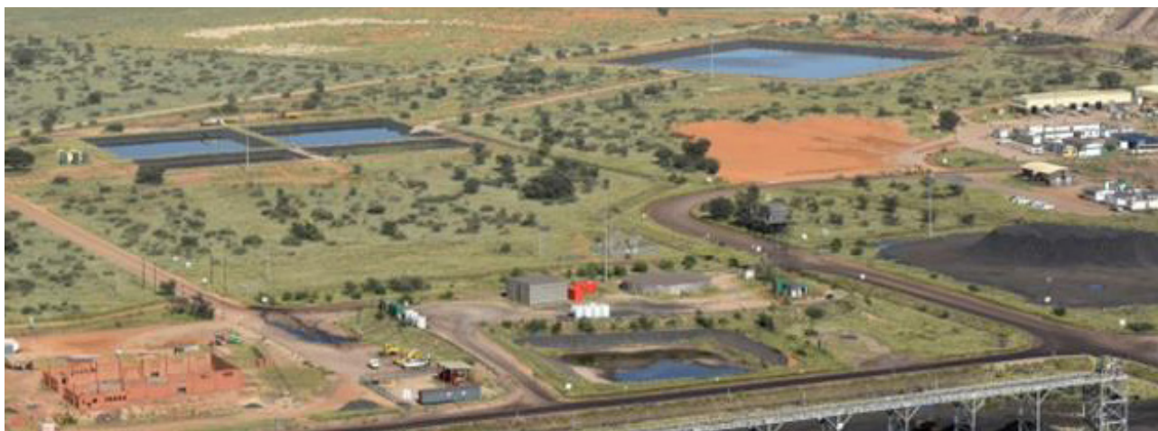
Figure 7: New storm water dam, with a 52,000m 3 capacity
