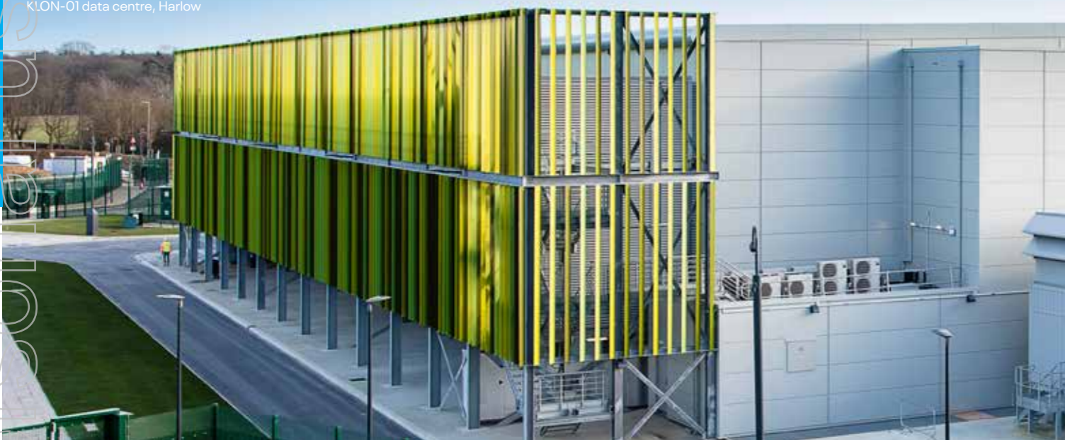
KLON-01 data centre, Harlow
