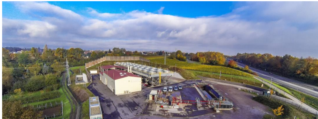
Vulcan Energy's 100% owned NatürLich Insheim, an operational geothermal renewable energy power plant in the Upper Rhine Valley, Germany.
