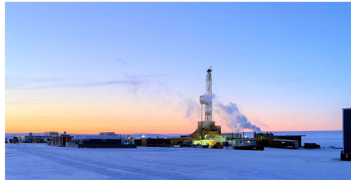
Arctic Fox rig onsite at Merlin-2
