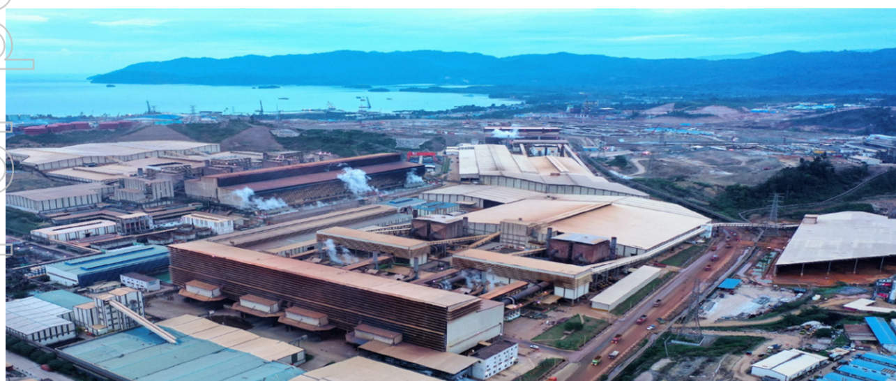
Hengjaya and Ranger RKEF operations
