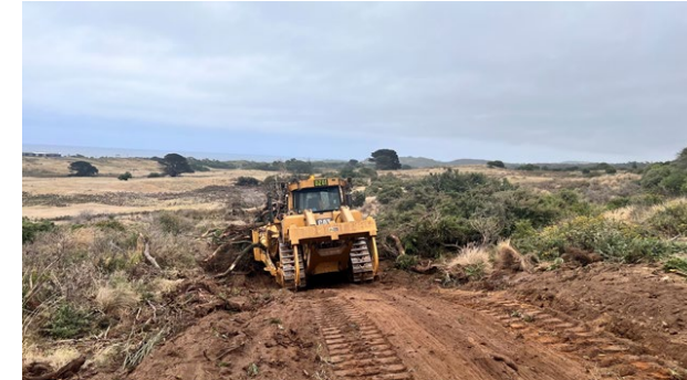
Commencement of earthworks – Jan 2022
