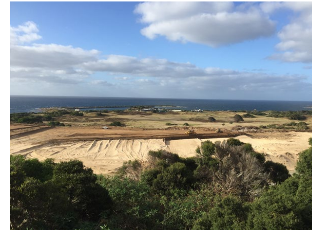
Earthworks Progress – Mid March
