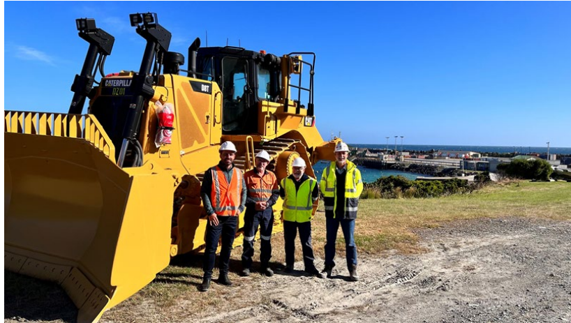
Dozer DZ01 arriving on site to start earthworks _ January 22
