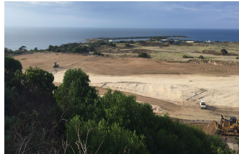
Process Plant Earthworks nearing completion_ March 22
