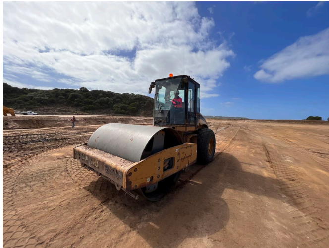
Compaction Rolling of Process Plant Area _ March 22
