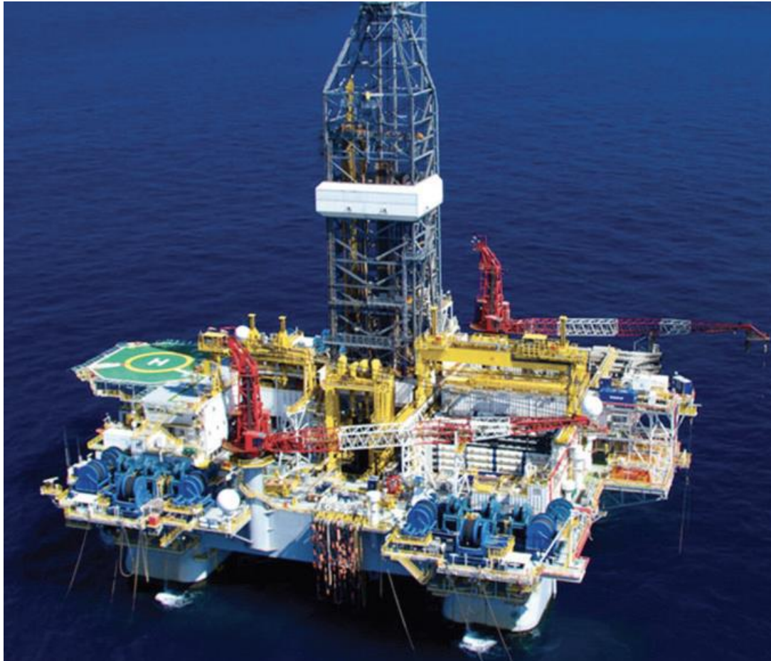
Valaris MS-1 Semi-Submersible Drill Rig
