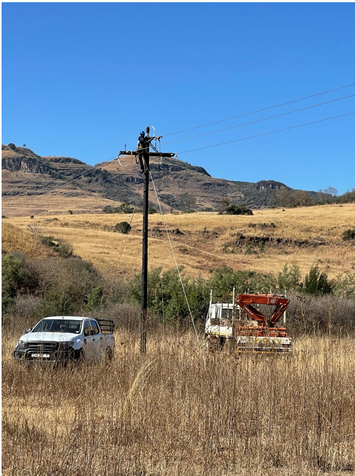
Figure 11– New power line installation across the Northern section of our Mining Rights (Close to Vaalhoek and Frankfort Mines.) The powerline will add to the required capacity for the new gold plant and extends from north to south over 20 km within the current Mining Rights area.
