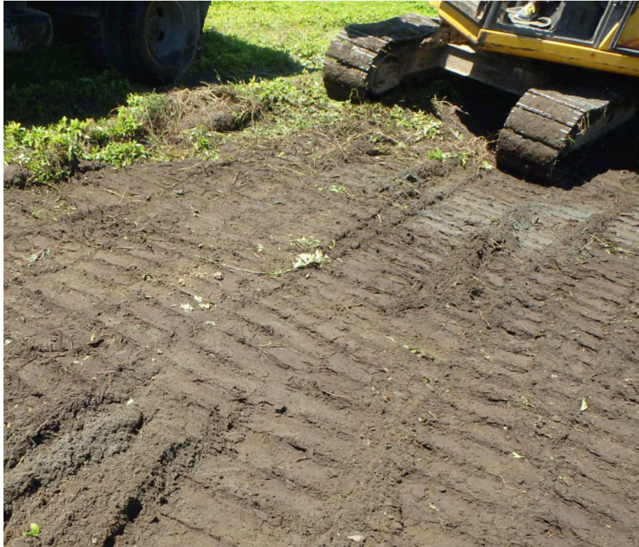
Plate 5 – Sampling site reclamation
