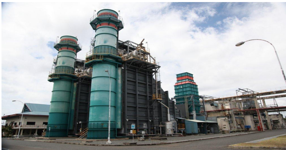
Sengkang Power Station in South Sulawesi, Indonesia
