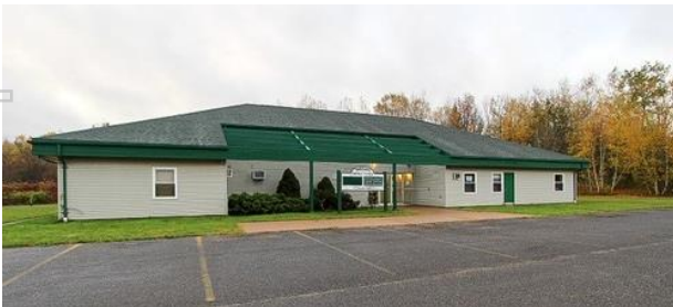
Treatment Facility in Nova Scotia
