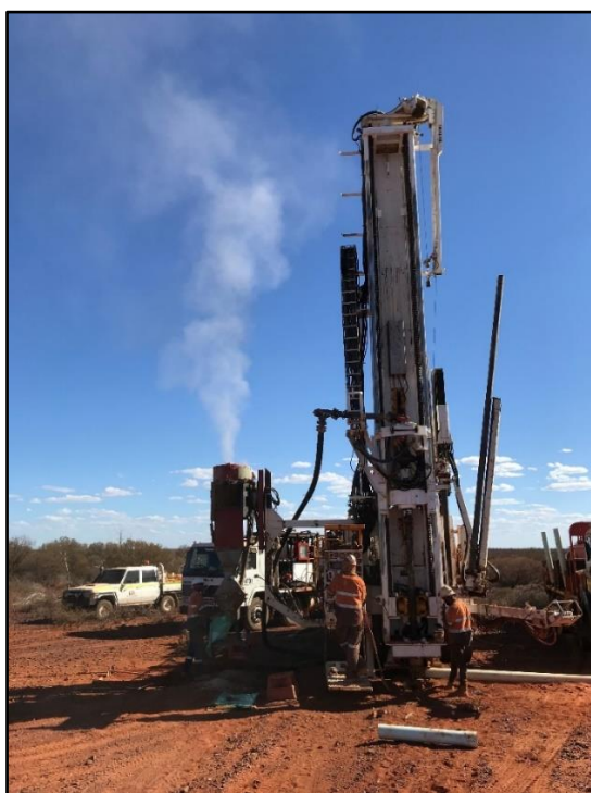
Image 1 – RC drill rig operating at the Earraheedy Project
