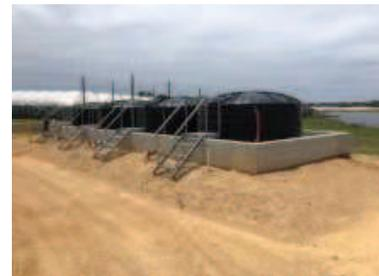
It is then pumped through a *Priva nutri-jet* managed fertigation system which features a mixing tank for soluble fertilisers and four storage tanks for dosing mixed solution. The mixed solution pumped to the plants using impellor pumps with variable speed drives. Pump sizes are typically 14KW or 22KW
