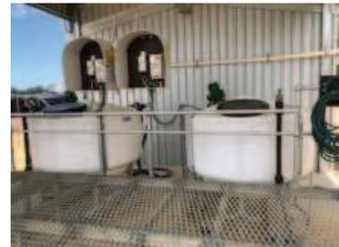
A *Netafim* radio net controller manages irrigation shifts. The water is delivered to the to the substrate plantings using pulse irrigation with typically shifts less than 10 minutes and delivering anywhere from 100 to 175 litres per second to the pots. On average two to three valves make-up a shift, which feed water through 20 to 30 laterals per valve.
