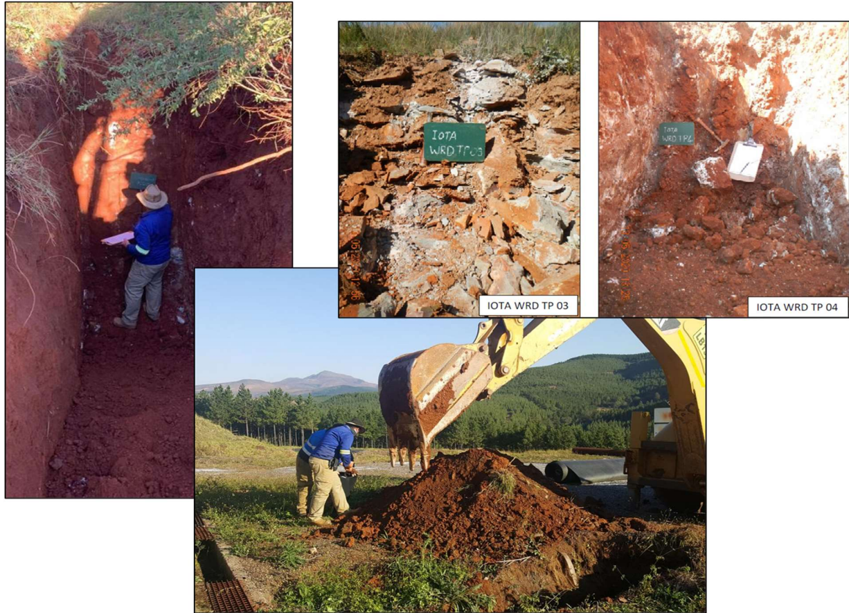
Figure 2: Test pits for ground stability
