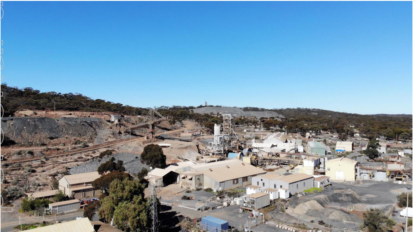
Existing Norseman Project administration and processing complex.
