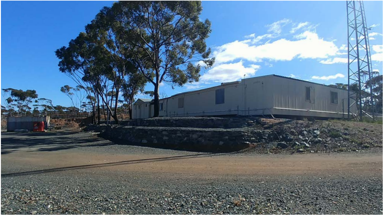
The OK Underground Mine Office and Changerooms, an example of the substantial existing infrastructure.
