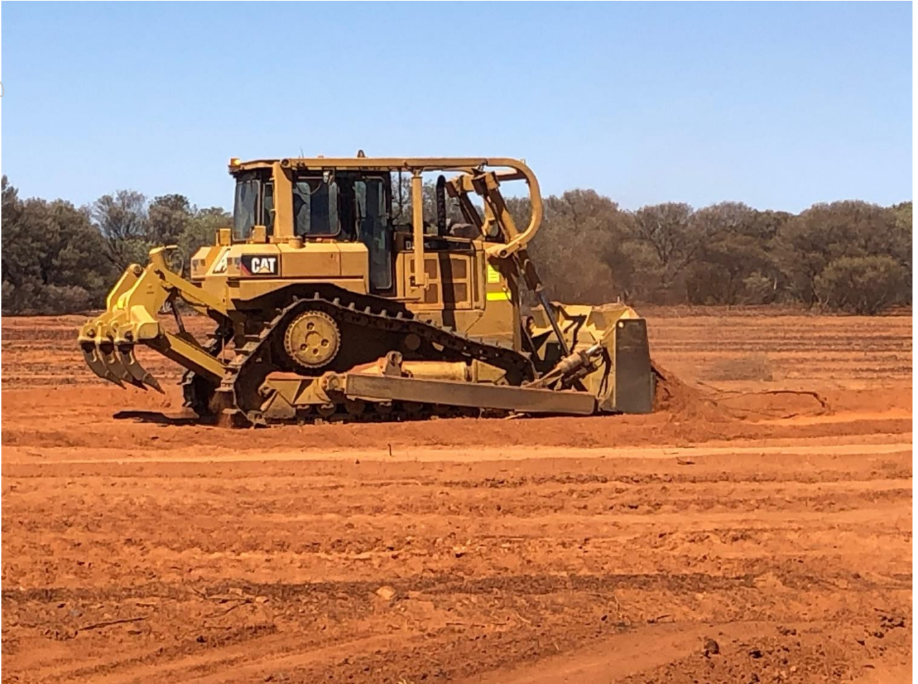
Topsoil stripping – Iron Ridge Project
