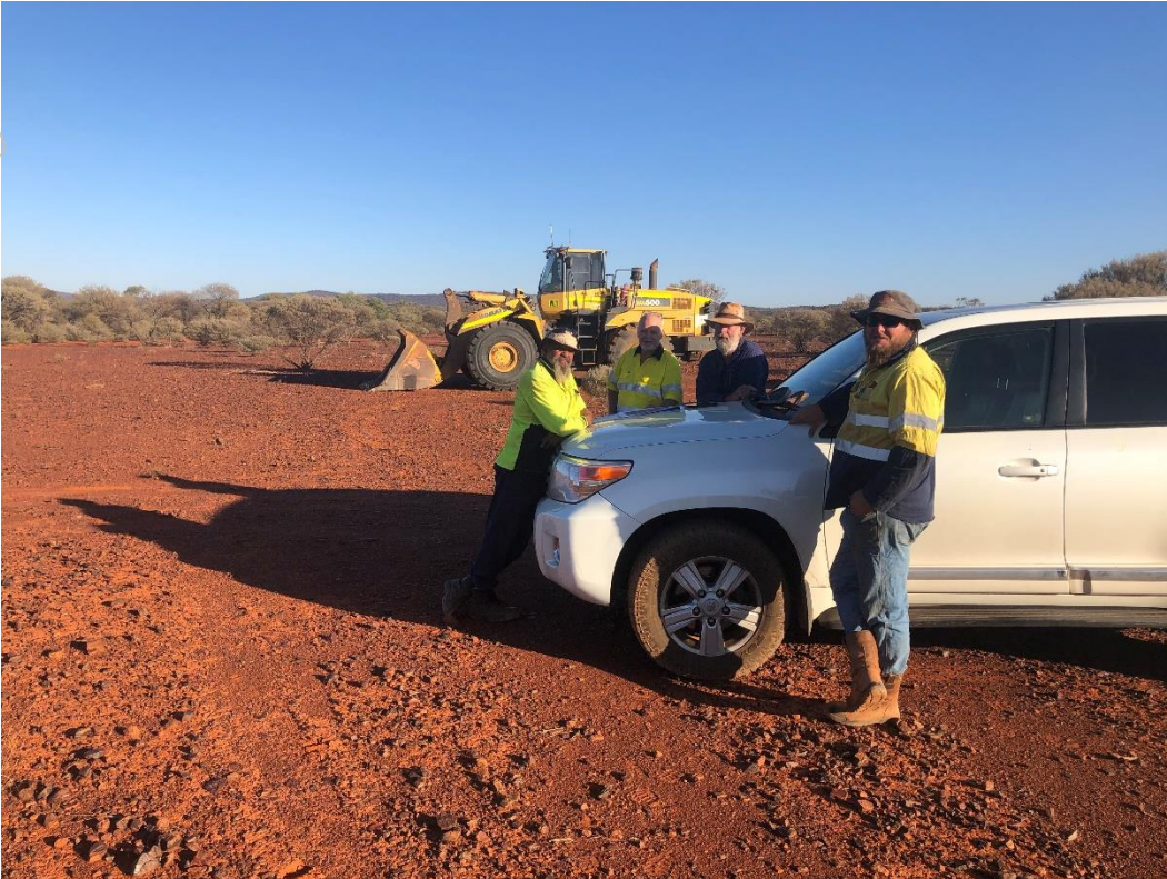
First pre-start meeting – Iron Ridge earthworks crew
