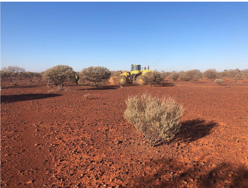
Clearing activities – Iron Ridge Project
