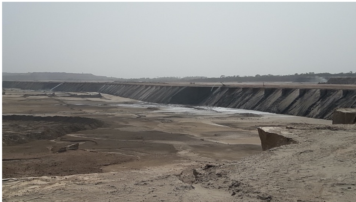
Figure 17: Morila Tailings Storage Facility showing hydraulic mining of upper layer of tailings to expose lower 'higher-grade' tailings
