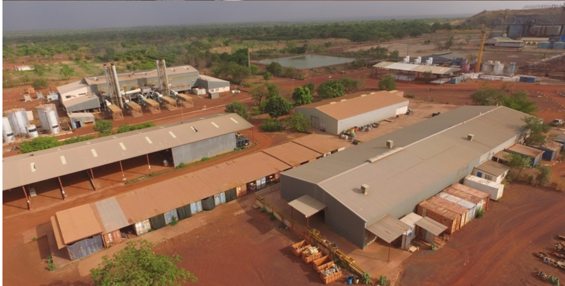
Figures 18-20: Photographs of the plant from top to bottom; Primary Crusher with processing plant in background, entrance to the plant area and aerial view of the warehousing sheds and power plant.
