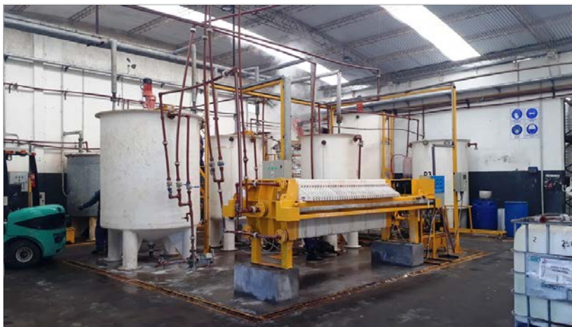
Figure 1. Rincon Lithium Project – Pilot Plant Lithium Carbonate Production Operations
