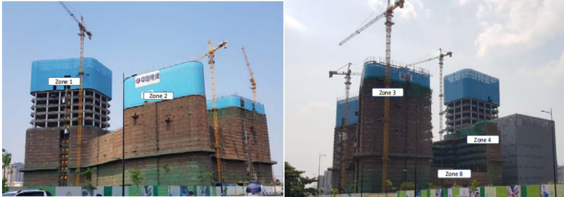
Installation of External Safety Net Protection - PPCC
