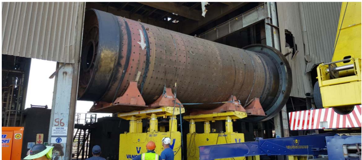
Figure 4: Mill Removal From Structure
