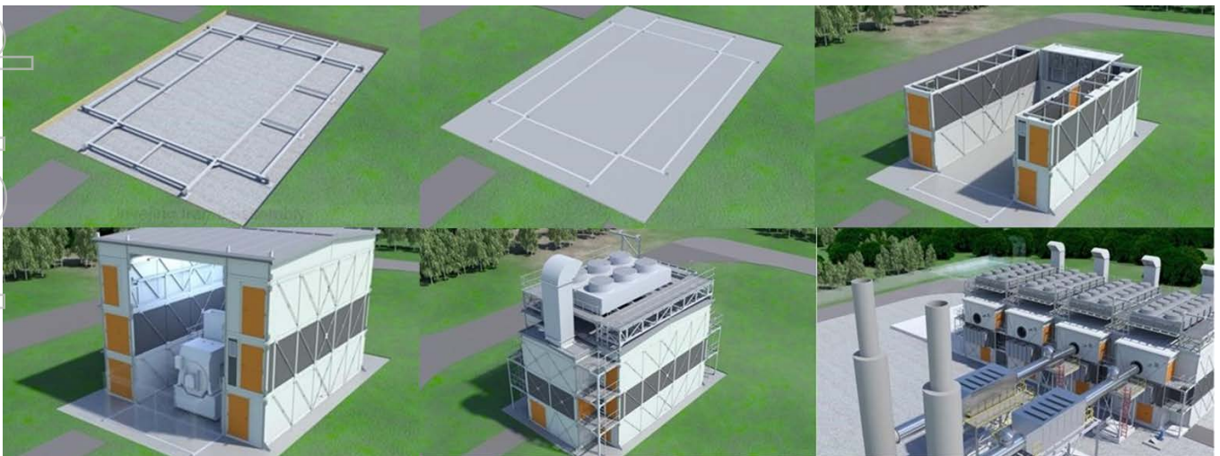
Figure 6: Syama Hybrid Power Plant – Wärtsilä Unit Modular Construction
