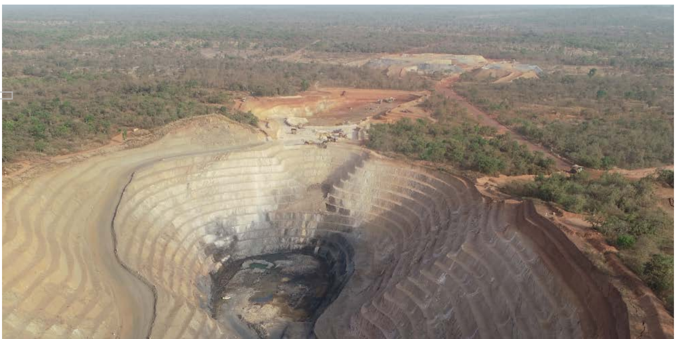
Figure 2: Northern end of the Namakan pit showing the commencement of the North pit in the background
