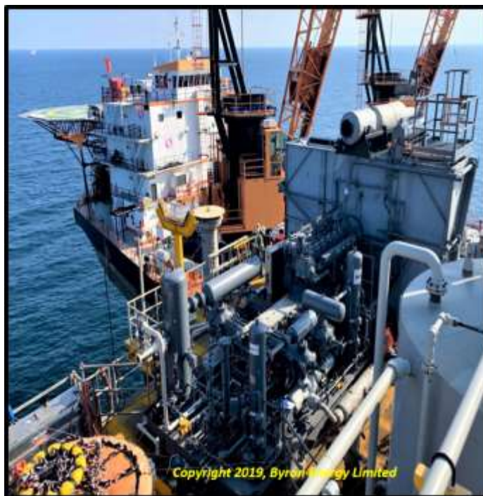
SM71 compressor upgrade construction spread
