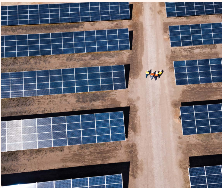
Darling Downs Solar Farm in Queensland
