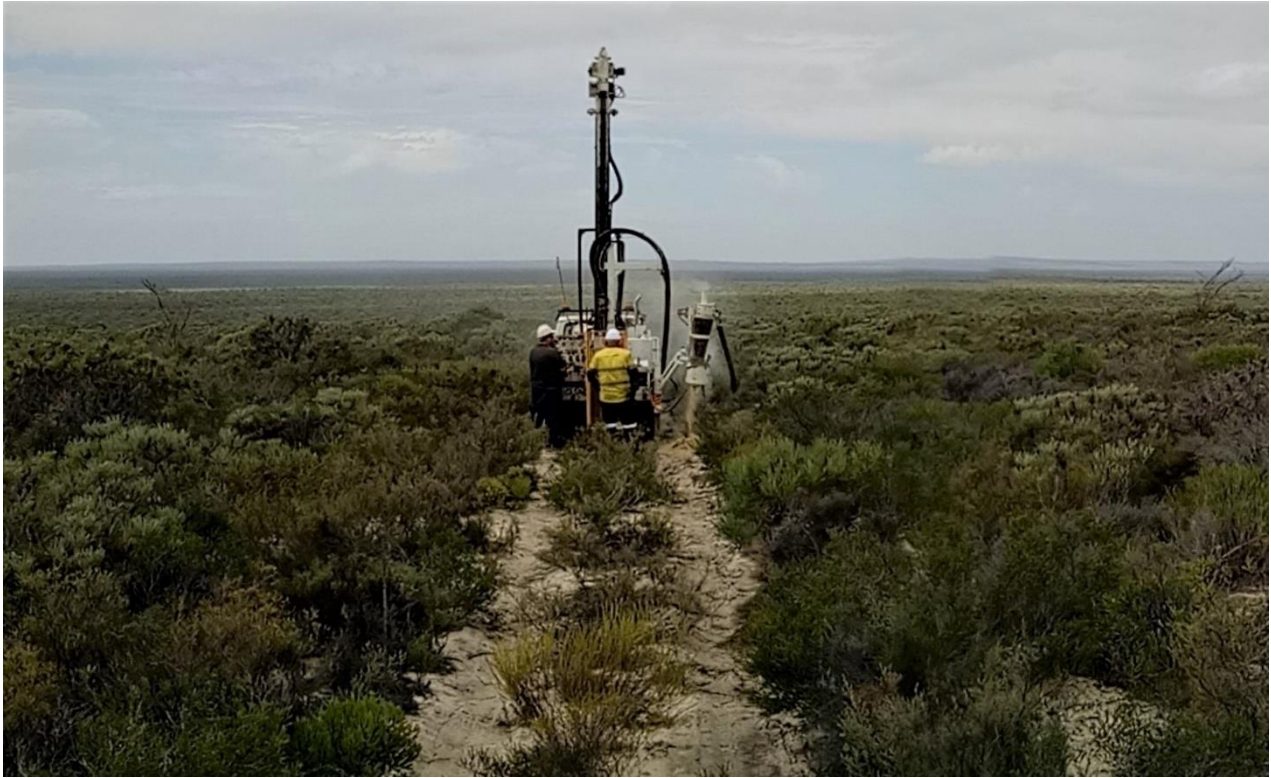
Figure 4: Landcruiser mounted Mantis 82 NQ sized aircore drill rig
