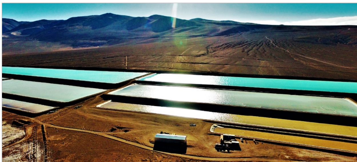
Figures 3 - 4. Rincon Lithium Project – Current Operational 38Ha Evaporation Ponds
