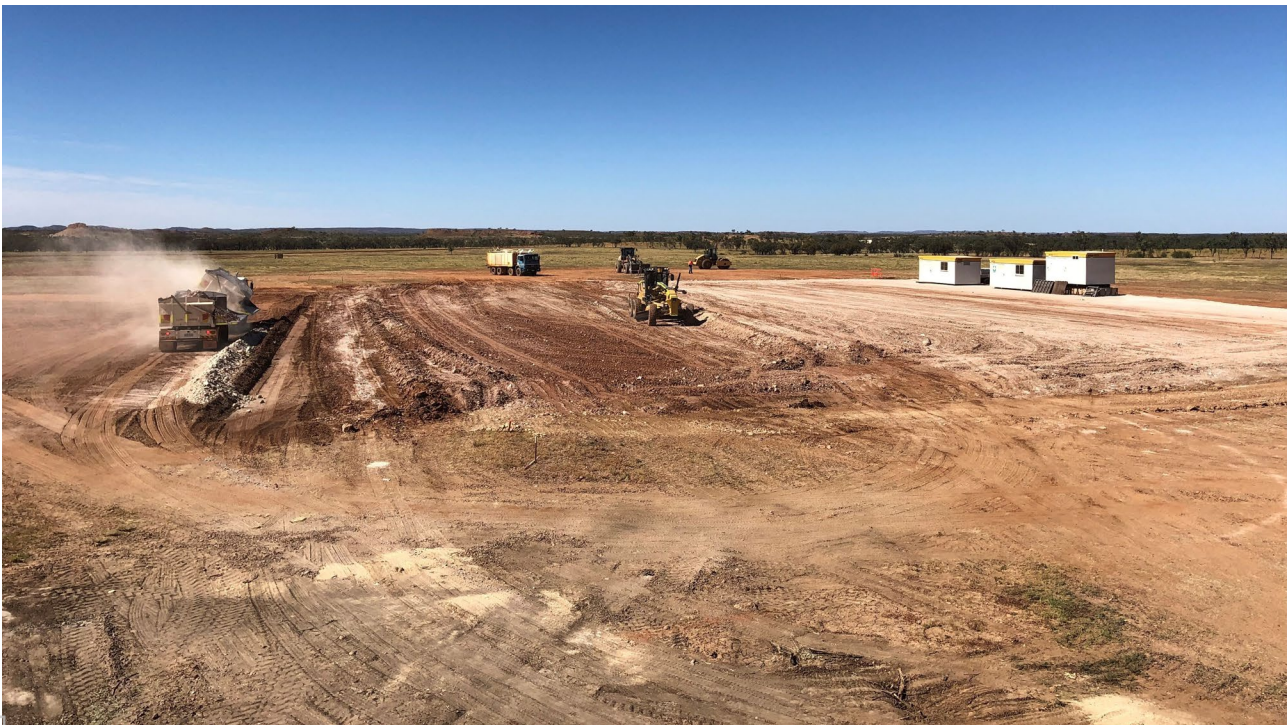
CAPTION: Earthworks commence at the Start-Up Plant location at Ardmore
