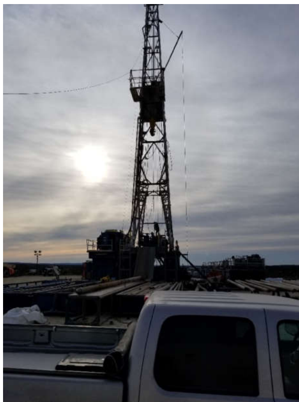
Drilling White Hat 20#3, East Permian Basin, Texas
