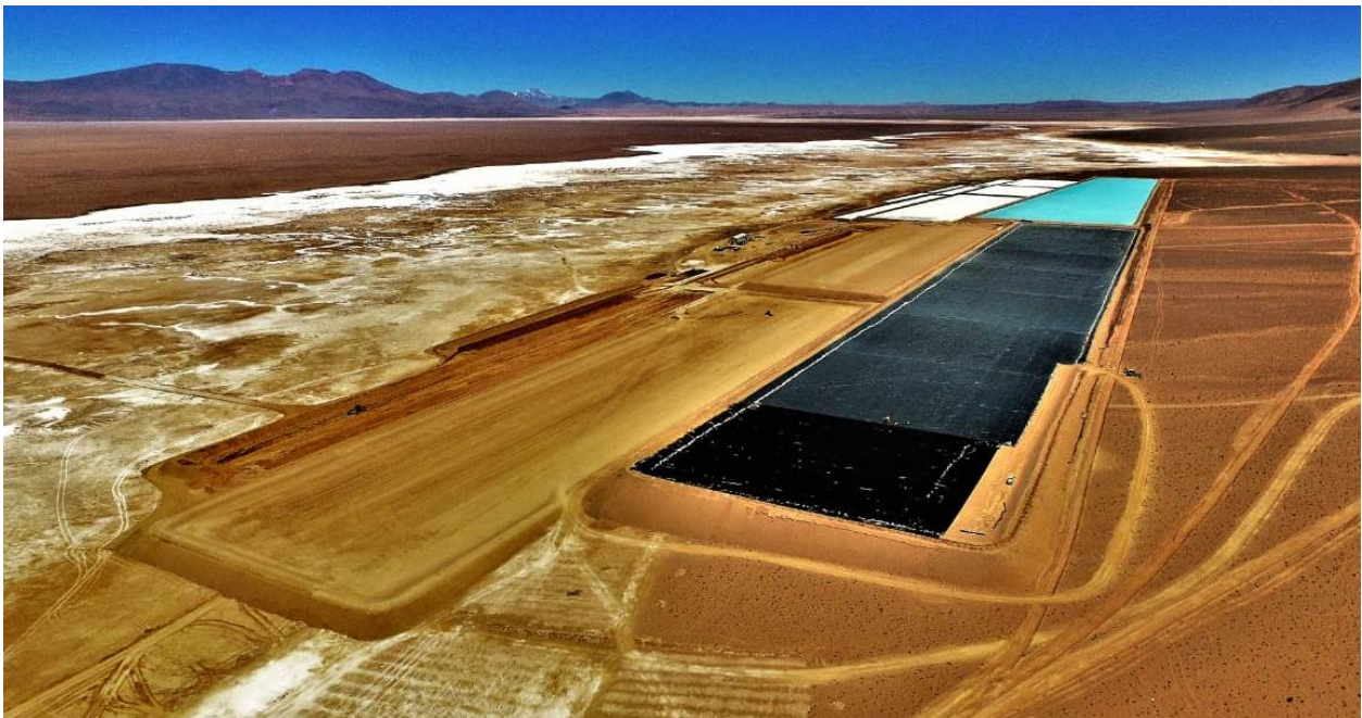
Figure 10: Stage 2 evaporation ponds with ongoing construction works
