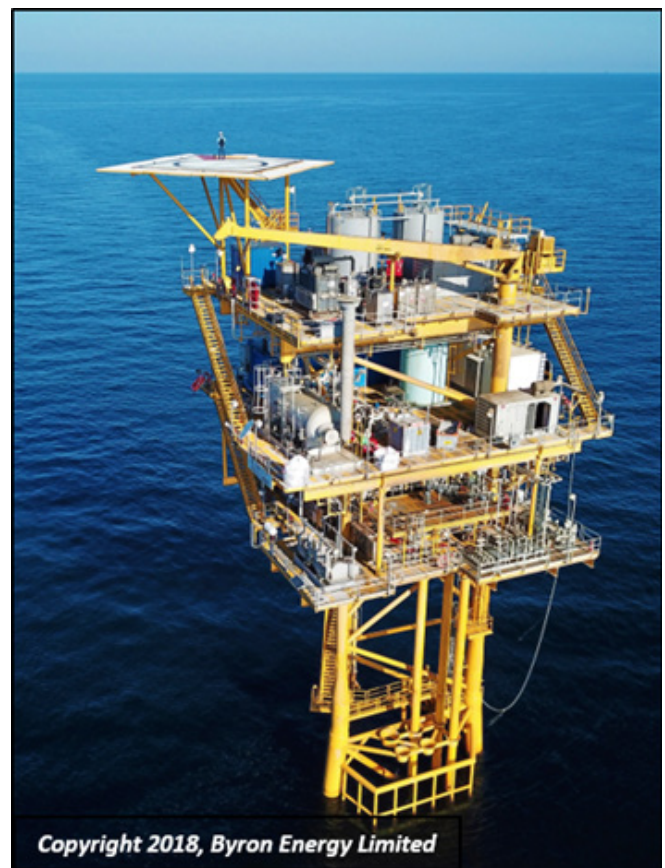
Copyright 2018, Byron Energy Limited Byron Energy Operated SM71 F Platform Gulf of Mexico USA 25 April 2018
