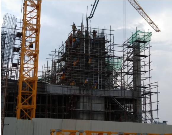
c) Activity work of casting concrete for Sprinkler Tank of ground floor (Zone-B)
