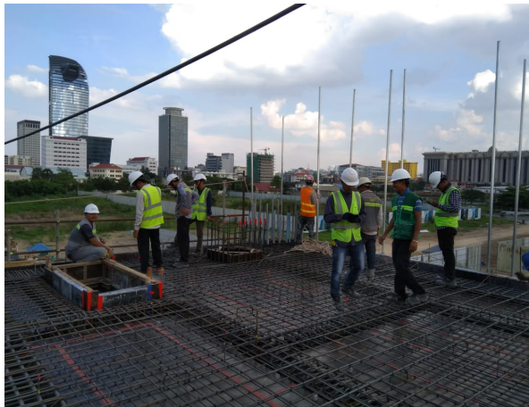
c) Activity work of casting concrete for Sprinkler Tank of ground floor (Zone-B)
