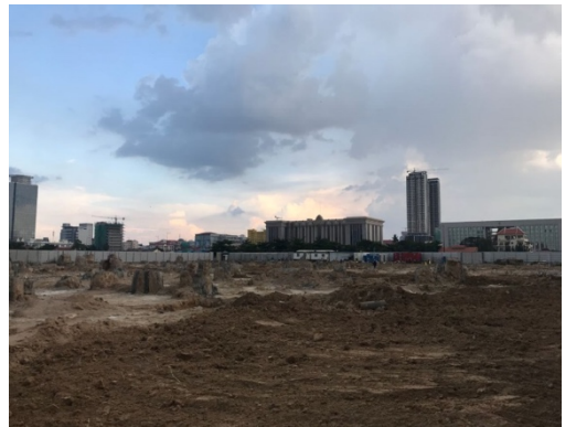
c) Re-install the boundary hoarding and leveling soil
