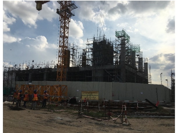
d) Activity work of installation rebars and formworks for 1 st floor slab and beam (Zone-B)
