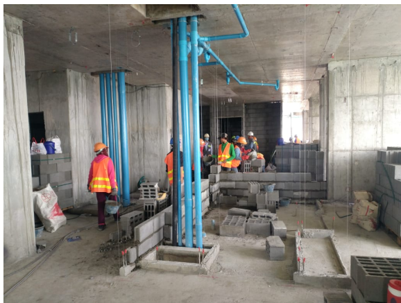
c) Brickwork for 11 th floor
