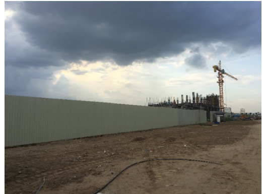
b) Re-install the boundary hoarding and leveling soil
