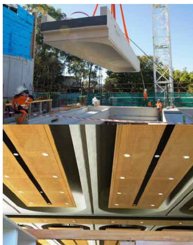
FIGURE 31 Queensland University's Global Institute Building – 33 precast EFC beams used in production
