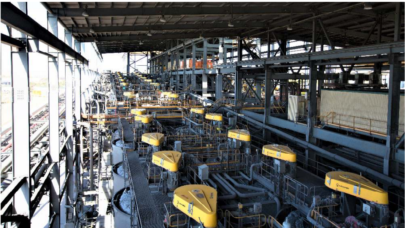
Figure 10: One of two flotation trains within the Century Processing Plant
