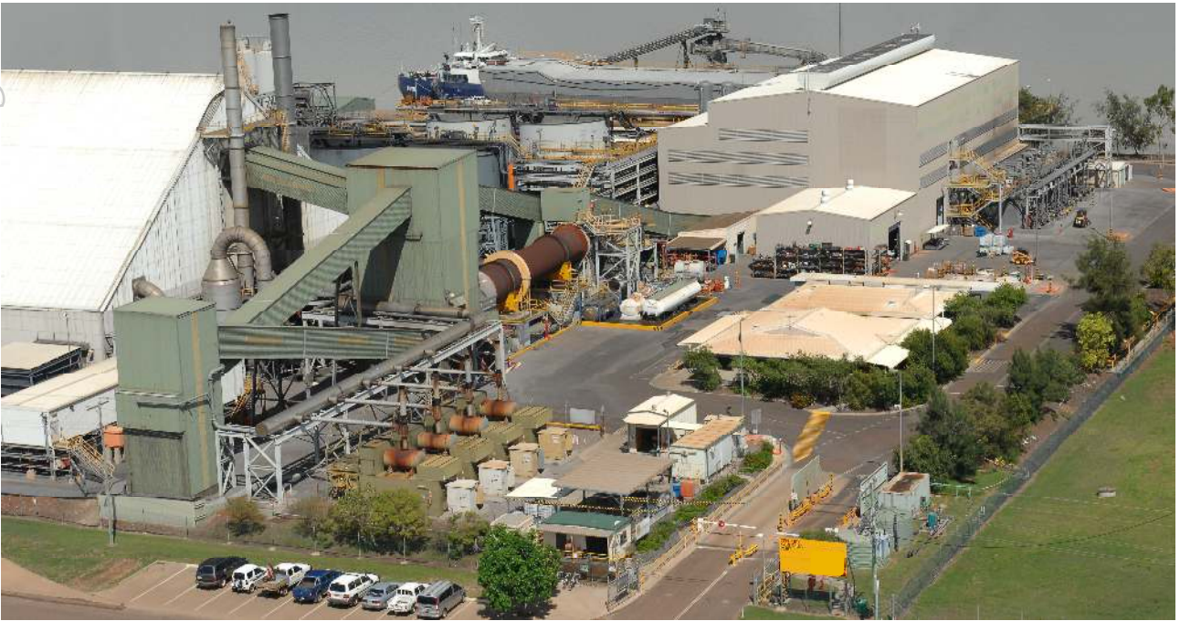
Figure 11: Karumba Port Facility
